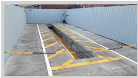
Anlaby Road on-site chassis wash
