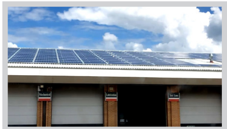
Reusable energy: Solar panels installed on the roof of Thames Travel depot in Didcot
