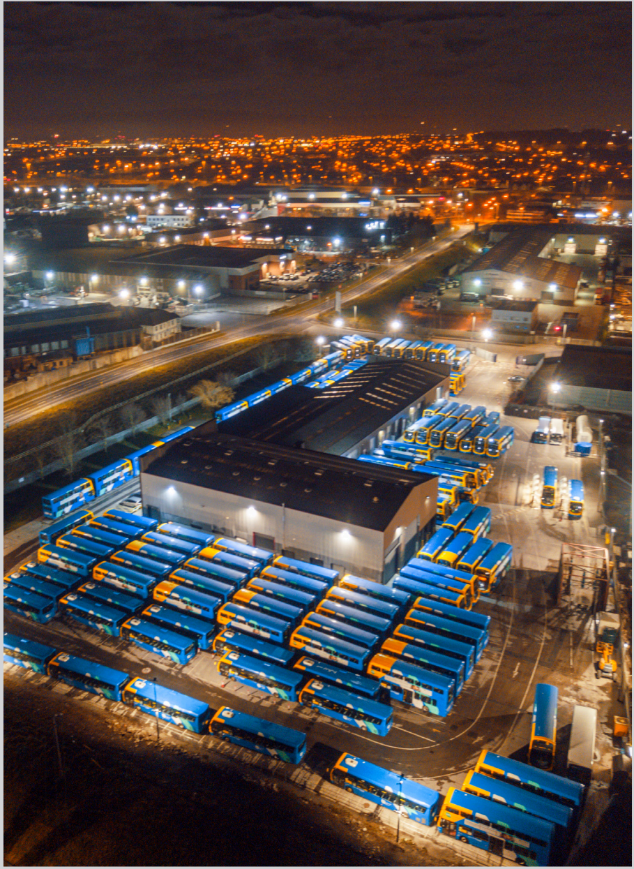
Ballymount depot: An aerial view of Ballymount depot at night.
