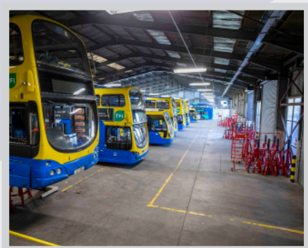
Ballymount workshop: Our workshop in Ballymount, where we will be installing electric charging points for buses.
