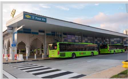
Alighting area at Pasir Ris Bus Interchange
