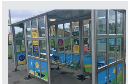
Purbeck Community Rail Partnership new bus shelter
