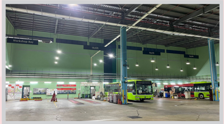
Energy-efficient LED lighting has been installed at the engineering workshop
