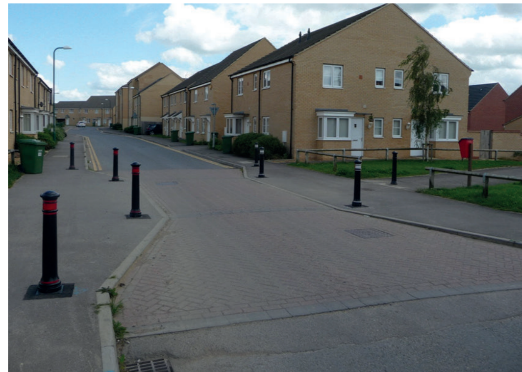
Fig. 8 Short single-track throttle at pedestrian crossing. Note the gentle ramp transition and good cross-visibility.
