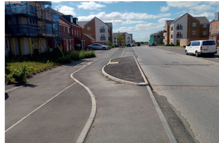
Fig. 34 Island Bus stop - This boarder is smaller than the minimum dimensions in LTN 01/20, and deflection on a 1.5m wide track is excessive. There is inadequate room to deploy a ramp or position a shelter. If space does not permit cycle segregation then alternative high quality provision should be made parallel to the main street.
