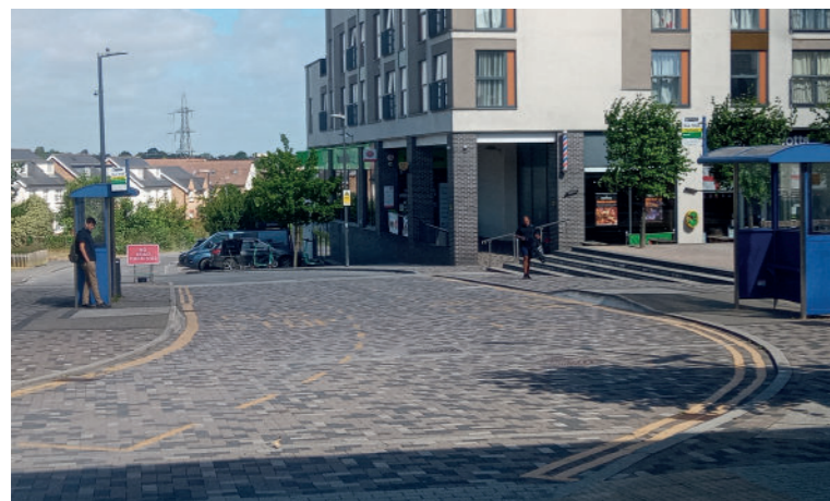
Fig. 13 Bristol Northern Fringe - Cheswick Village. This pair of stops in a shared space local square presents significant hazards. A stopped bus is likely to block the vehicular carriageway entirely. Note the treatment of boarders which involves excessively steep transitions to a 180mm high boarder only 2m long. The vehicular carriageway, is demarcated, but the approach intentionally uses colour to add ambiguity and blend the carriageway visually with the wider public realm.
