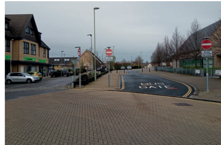
Fig. 9 Andover, East Anton Buses remain on a direct alignment on the primary street. Permeability remains for general traffic via a much more complex and circuitous route.
