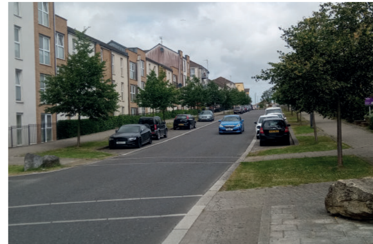
Fig. 1 Charlton Boulevard, Charlton Hayes, South Gloucestershire. The ideal solution for bus: a direct bus route with clear carriageways. Bus gates are anticipated at the top and bottom of the street.
