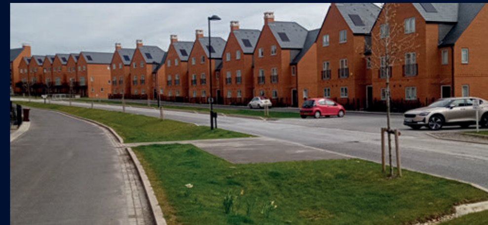
Fig. 14 The site of a future bus stop, with generous dimensions. This bridges a substantial swale feature. These must always be considered at the earliest stage of the s38 design and approval process.
