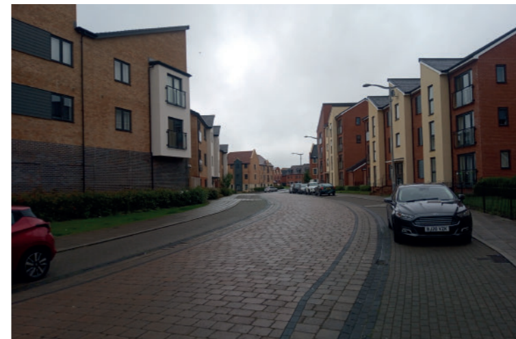
Fig. 10 Approach to surface treatment appears to narrow the carriageway, while allowing for tracking of larger vehicles.
