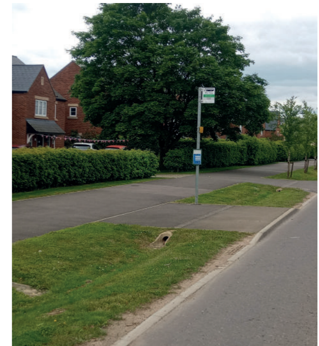
Fig. 40 The bus stop boarder needs to allow the swale to perform its drainage function effectively, while facilitating safe boarding and alighting for all users. Robustness and maintainability are key areas of concern.
