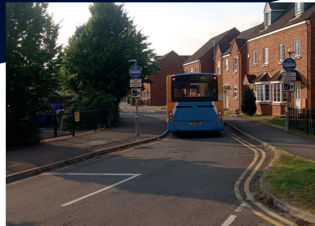
Fig. 19 Gloucester, Kingsway bus gate - One of three all of which involve CCTV enforcement. This is simple, robust, and extremely cost effective, especially since decriminalisation of moving traffic offences is now straightforward for Local Authorities to secure. Private enforcement can be an option.
