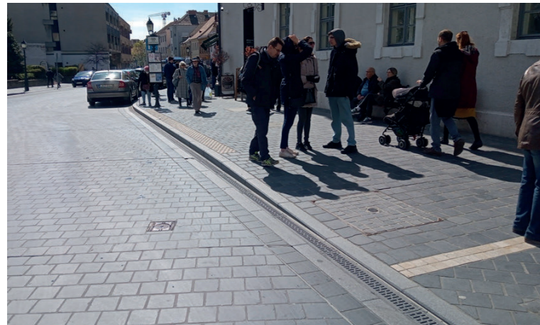
Fig. 12 Buda, Szent Haromsag Tere - A particularly sensitive approach to a busy stop in a shared space area. The edge of the vehicular area is clearly defined, with a 25mm upstand and contrasting colour kerb. The bus stop boarder has a full height kerb, gentle transitions and proper use of tactile edge markings.
