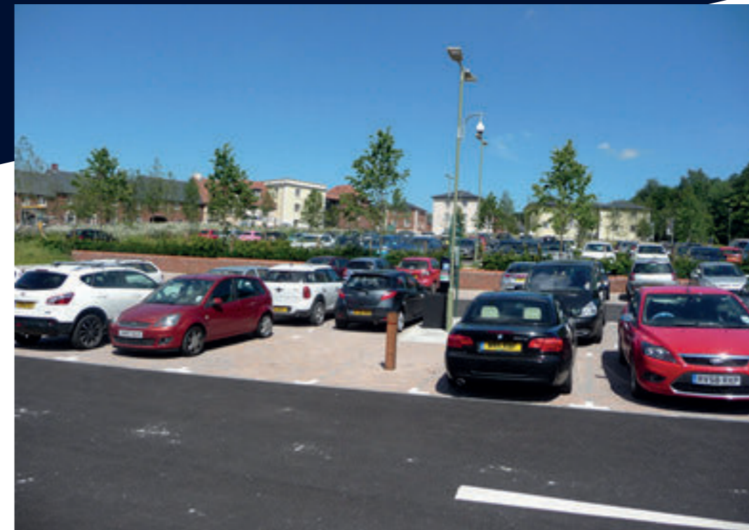
Fig. 22 Pitt Park and Ride - Permeable paving and generous planting help integrate the facility into a residential setting.
