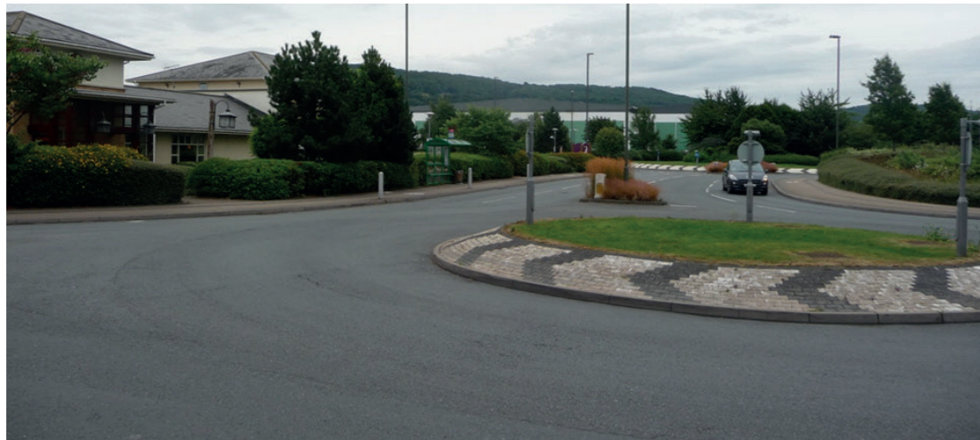
Fig. 18 Gloucester Business Park. A short double run into a busy mixed use development.
