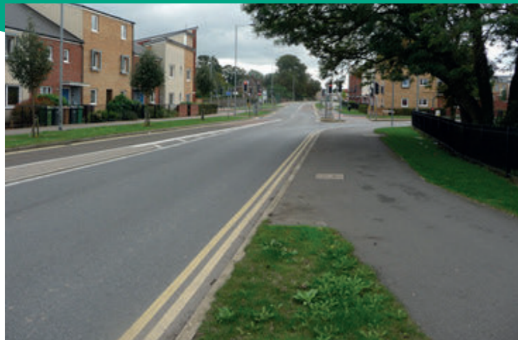
Fig. 20 Peterborough A15 London Road - Two alternating contra flow bus lanes. Approaching general traffic is merging back in from the right, with the approaching bus lane section in the distance. Among other things this imaginative approach saved substantially on construction costs.
