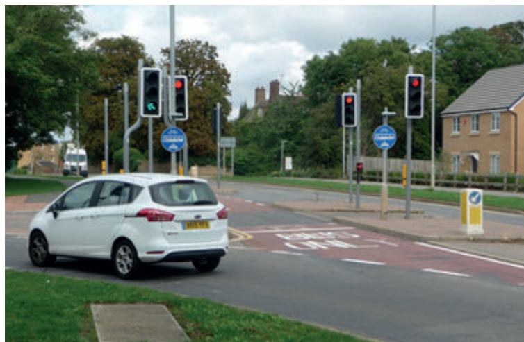
Fig. 21 Peterborough A15 London Road - Contraflow bus lane. With-flow general traffic is made to divert substantially offline behind the frontage on the left side of this picture.
