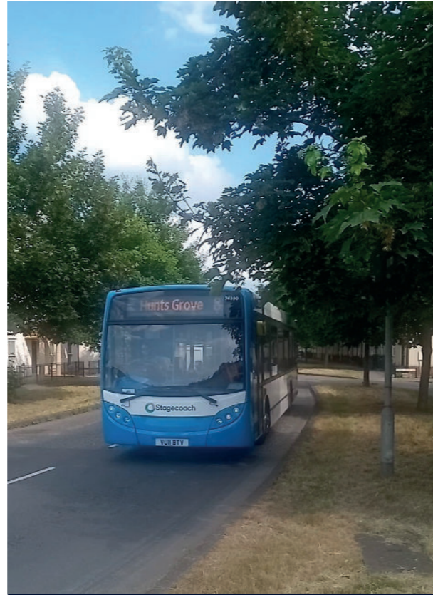
Fig. 41 Gloucester, Coopers Edge - A generous planting margin incorporating swales allows street trees to mature without affecting passing buses.
