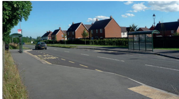
Fig. 37 Amesbury, Stockport Way - Partial pull-in at a bus stop on a major through route on the edge of a major urban extension, with a 40mph speed limit. While on residential streets on-carriageway stops are generally entirely acceptable, there is no “in-principle” operator objection to lay-bys. In fact, in certain cases they are necessary to support traffic flow and for safety.
