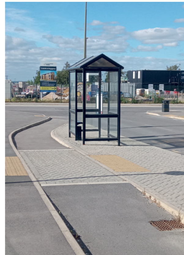
Fig. 35 Island bus stop - Within the same LPA and locality, this island stop is much more generous, with LTN01/20 compliant dimensions. A cantilever shelter backing onto the track would allow disabled users to enter, and provide a level of protection on the back edge. Attention to detail is of the essence, putting the designer in the position of users.
