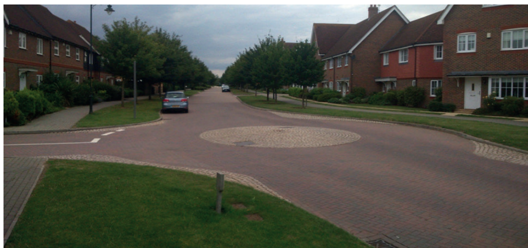
Fig. 6 Mini-roundabout and overrun feature calms traffic by occasional introduction of a feature obstacle. These should be tracked for 12m buses.
