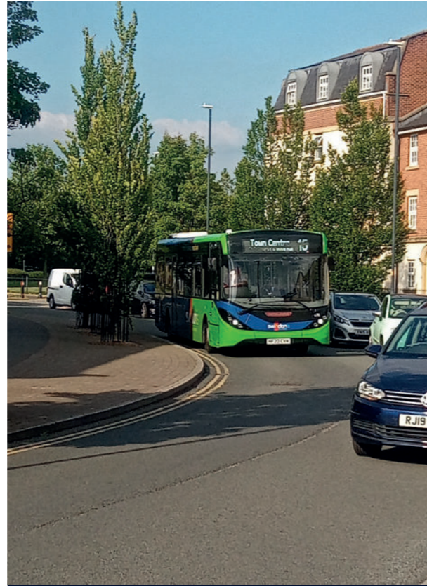
Fig. 47 This length of primary street, at 6.5m wide, permits parking on one side its whole length. High density and continuous frontage, with limited parking provision typically causes acute parking pressure on-street. After 5pm the street is effectively reduced to single carriageway for long distances.
