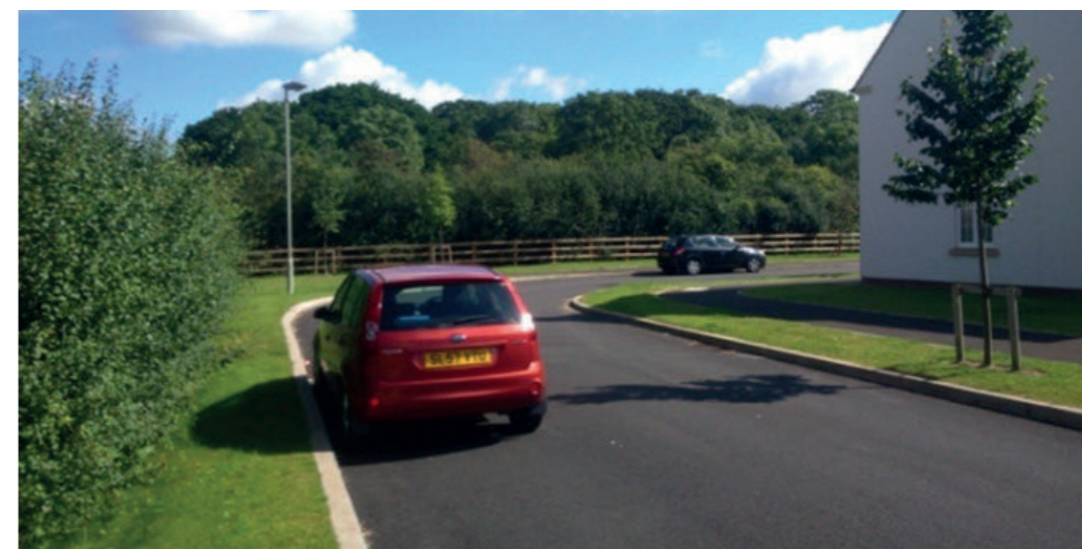
Fig. 3 Tight bends and limited visibility, combined with 6m width and uncontrolled on street parking means this road is not suitable for bus operation.
