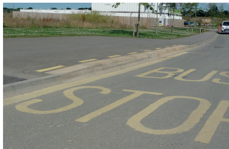
Fig. 32 Andover, East Anton MDA - Preferred 160mm raised boarder detail. DfT Inclusive Mobility guidance (Jan 2023) offers further important advice.
