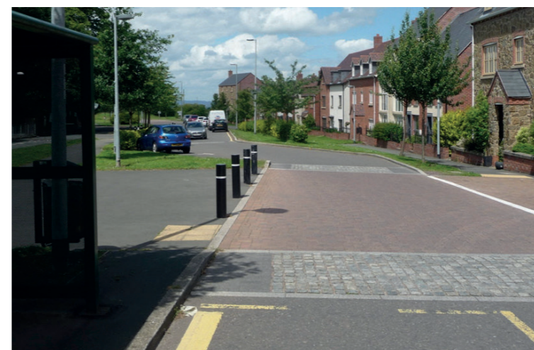
Fig. 11 Telford Lawley phase 1 - Careful use of offsets, changes in width and surface, and controlled on-street parking are used to create visual interest and reduce speeds while avoiding delay to buses.
