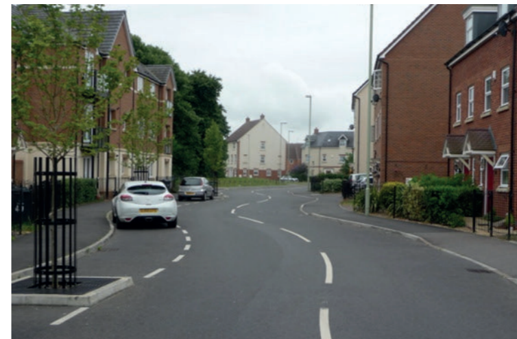
Fig. 2 Unnecessary deflection. This street was intended for use by buses but this has proved impractical. Just two or three cars parked on-street, make tracking effectively impossible for buses.
